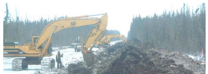
Figure 12: Backfilling After Lowering-in
