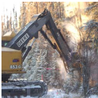
Figure 10: Clearing Timber from the RoW
