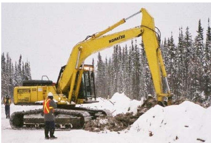
Figure 4: Construct Field Verification (test pits)
