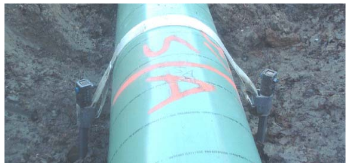
Figure 8: Screw Anchor Installed in a Dry Ditch
